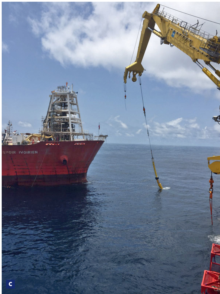
C Production riser replacement
