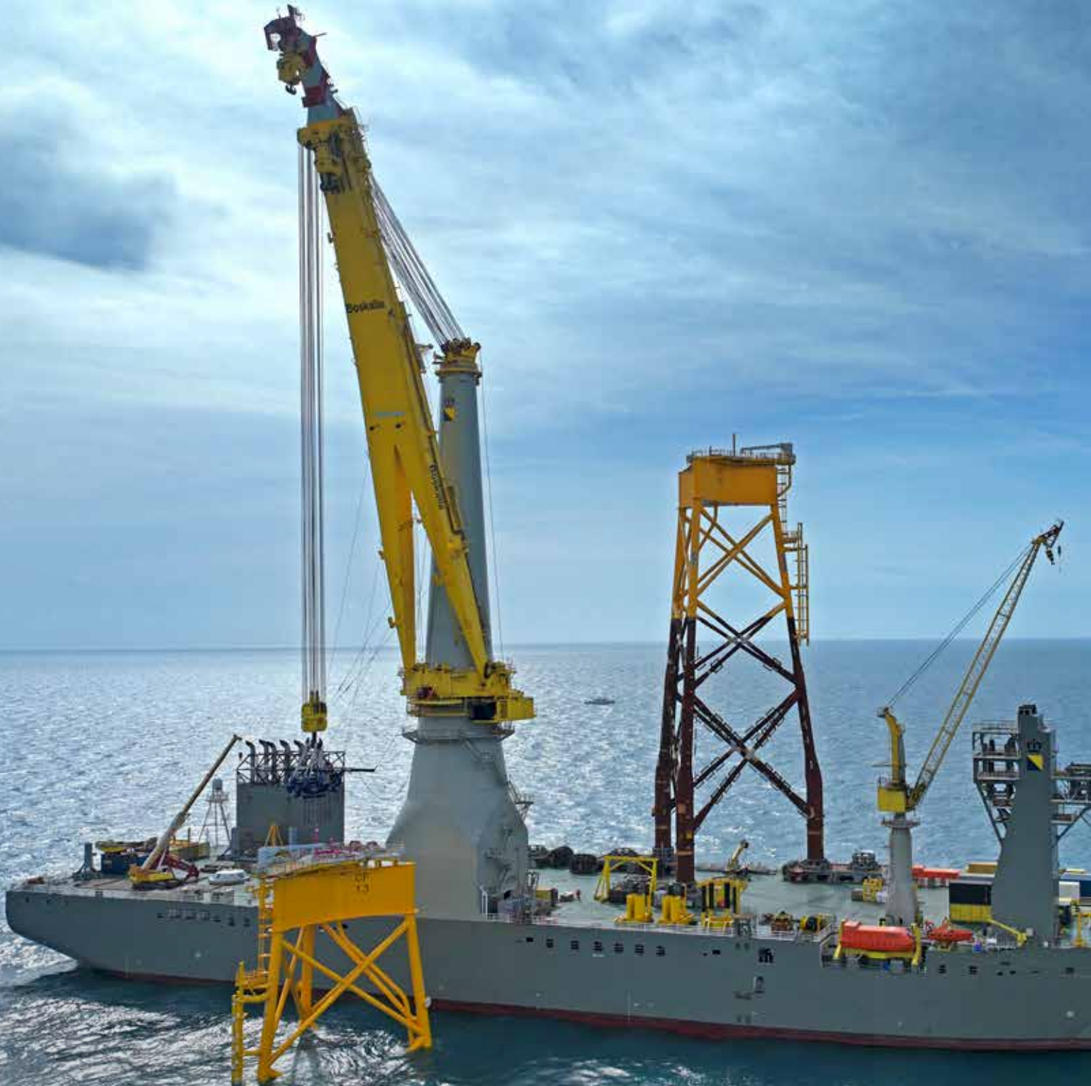
The Bokalift 2 crane vessel installs wind turbine foundations in Taiwan
