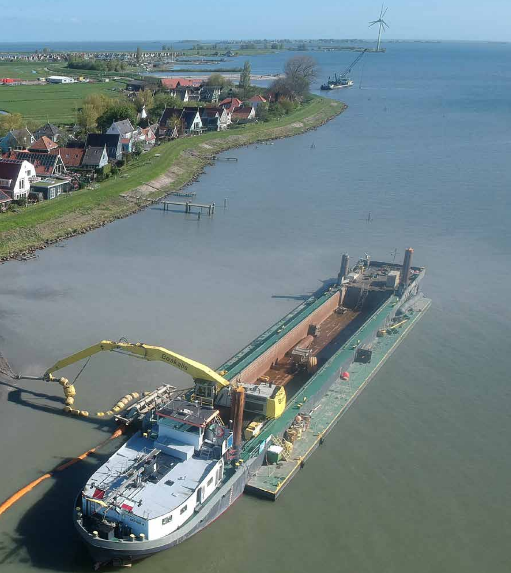
Dike reinforcement work as part of the Markermeerdijken project, the Netherlands
