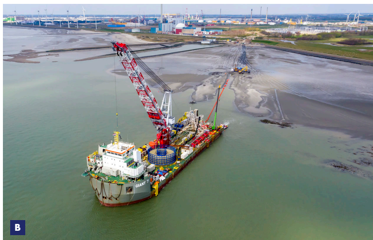
A Schematic of cable route with in yellow the shallow parts/sandbanks B Cable Lay Barge Giant 7 during the shore pull-in
