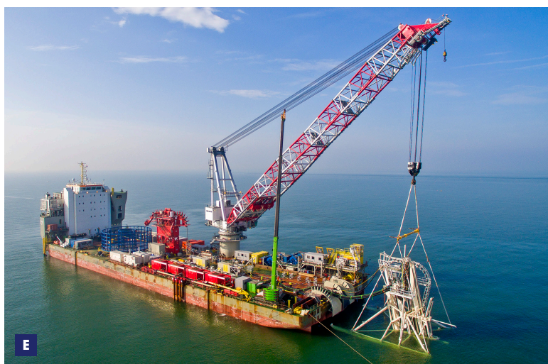
C Cable Lay Vessel Ndurance during the 2 nd end platform pull-in
